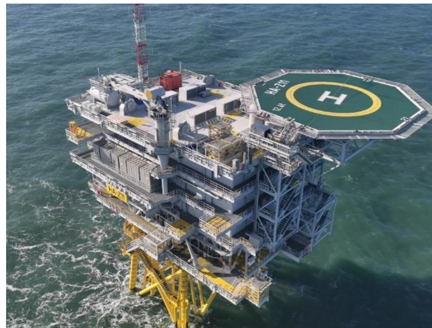
Figure 32 One of the fixed offshore substations used at the Hornsea One project. Image courtesy of Ørsted. All rights reserved.
