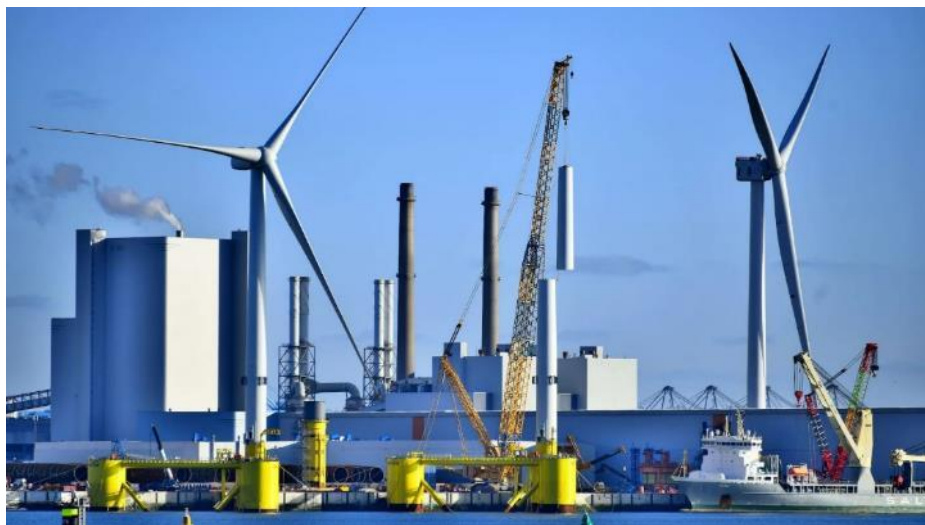
Figure 41 Floating offshore wind turbine final assembly taking place at port. Photo of the Kincardine Offshore Wind Farm project courtesy of Principle Power.
