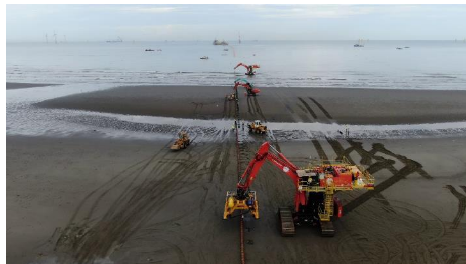
Figure 36 Offshore array cables installed at landfall. Image courtesy of Jan de Nul. All rights reserved.
