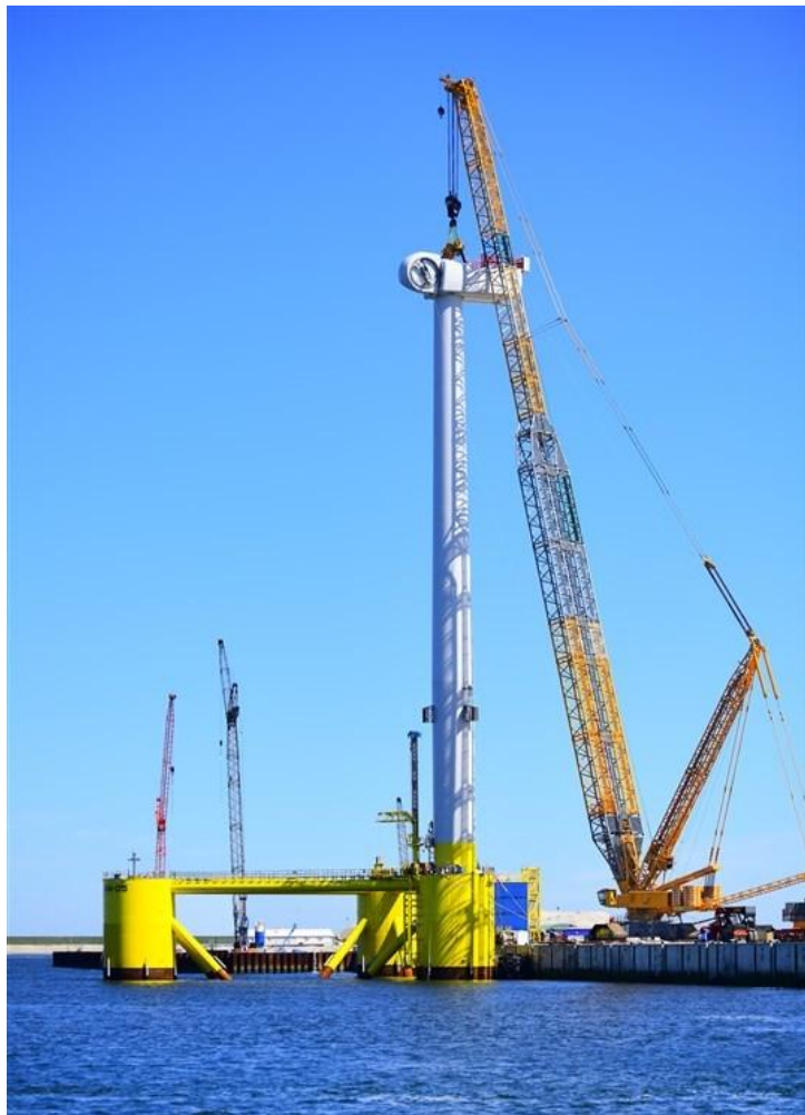
Figure 42 A landside crawler crane lifting a nacelle onto a floating substructure. Image courtesy of Port Pictures / Danny Cornelissen. All rights reserved.
