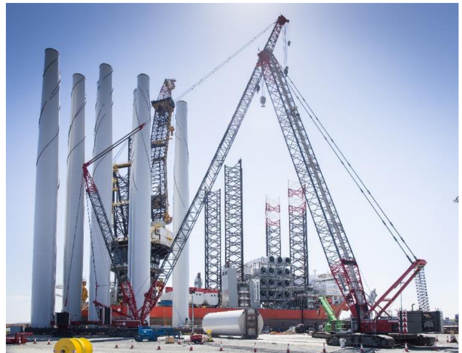
Figure 16 Offshore wind turbine towers being stored at the quayside of a port. Image courtesy of TMS. All rights reserved.
