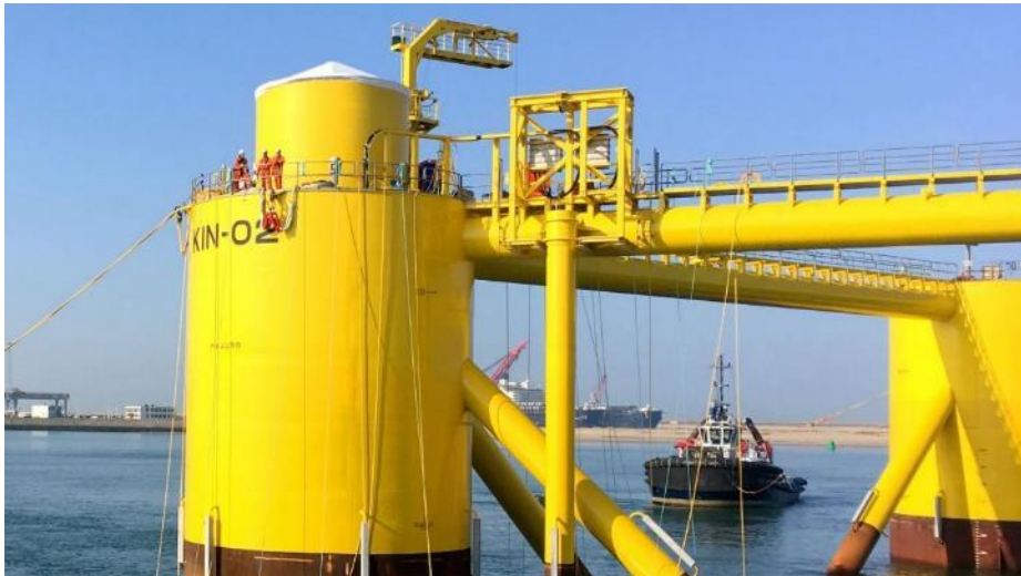
Figure 26 Secondary steel elements on the floating substructures used at the Kincardine project. Photo of the Kincardine Offshore Wind Farm project courtesy of Principle Power.
