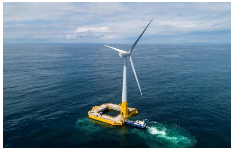
Figure 2 Example of a barge floating substructure. Image courtesy of BW Ideol. All rights reserved.
