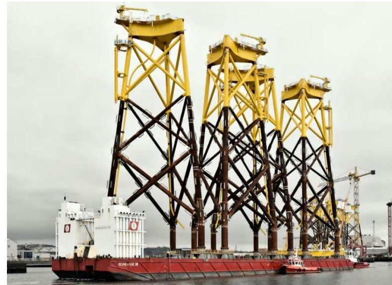
Figure 11 Example of jacket foundations being transported.
