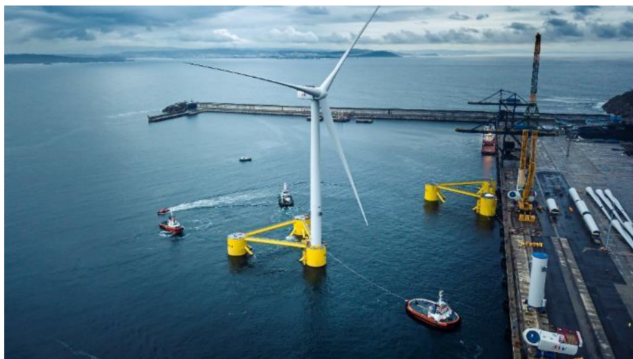
Figure 43 An assembled floating offshore wind turbine starting its tow-out for the WindFloat Atlantic project. Photo of the WindFloat Atlantic project courtesy of Principle Power/Ocean Winds.
