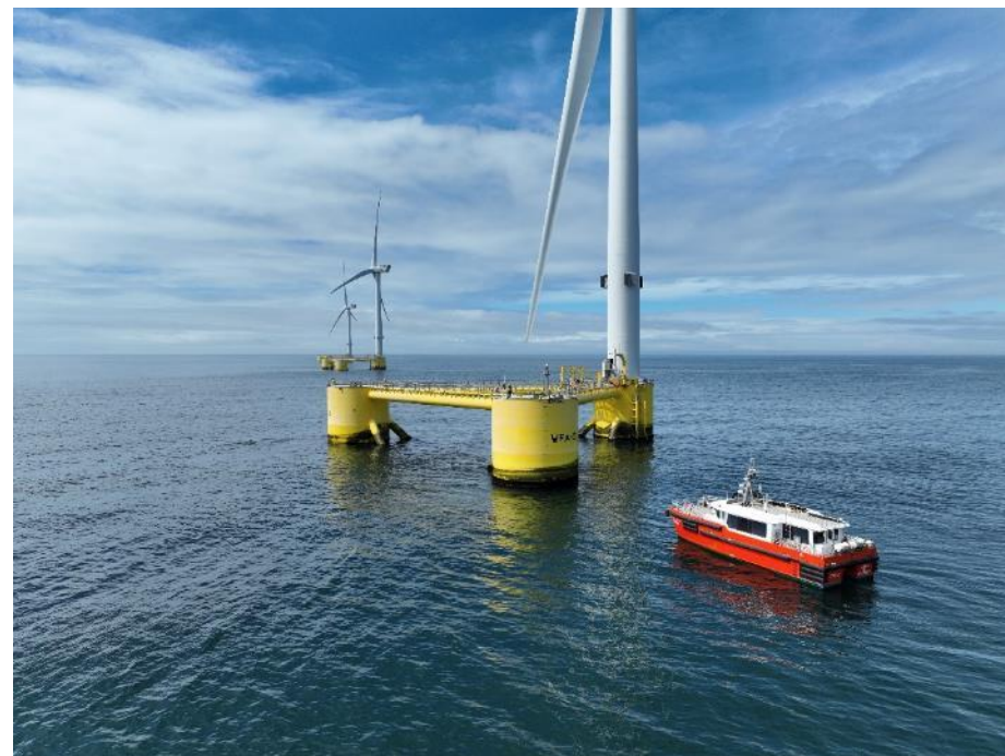
Figure 47 A crew transfer vessel servicing the WindFloat Atlantic floating offshore wind farm. Photo of the WindFloat Atlantic project courtesy of Principle Power/Ocean Winds.
