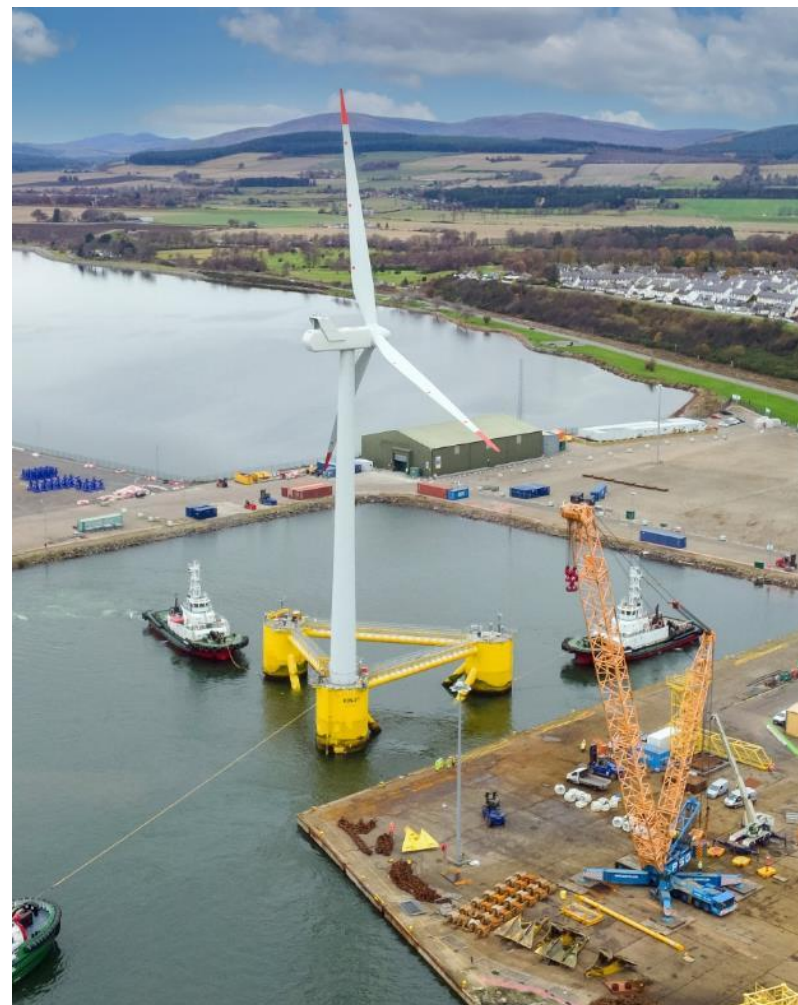
Figure 44 The Port of Cromarty Firth used as the construction port for part of the Kincardine project. Image courtesy of Port of Cromarty Firth. All rights reserved.
