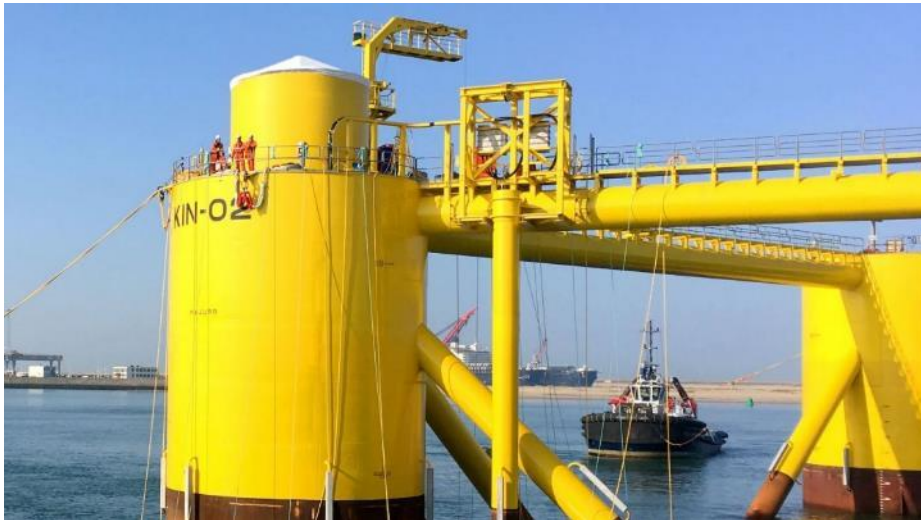
Figure 24 Secondary steel elements on the floating substructures used at the Kincardine project. Photo of the Kincardine Offshore Wind Farm project courtesy of Principle Power.
