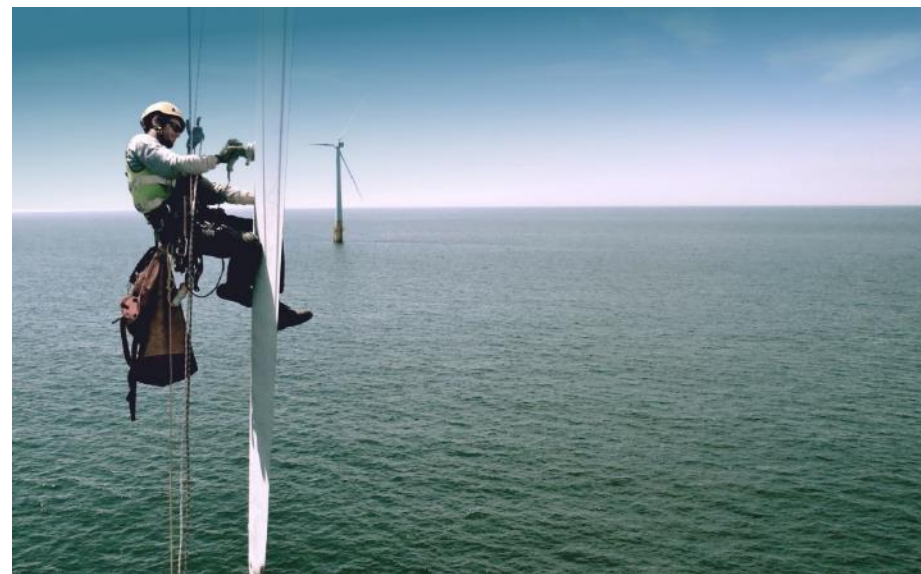
Figure 43 Blade inspection and minor repair being carried out by a rope-access technician. Image courtesy of Altitec. All rights reserved.
