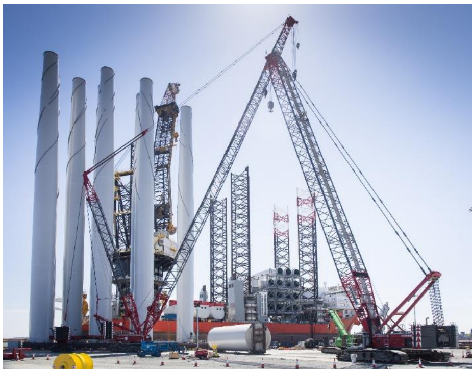
Figure 14 Offshore wind turbine towers being stored at the quayside of a port. Image courtesy of TMS. All rights reserved.
