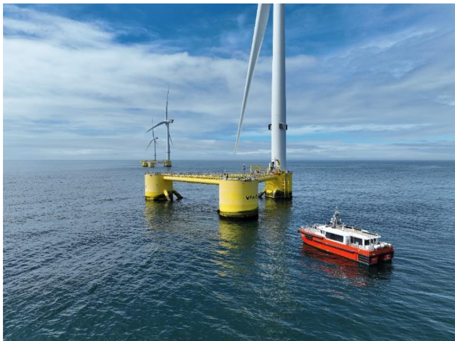
Figure 45 A crew transfer vessel servicing the WindFloat Atlantic floating offshore wind farm. Photo of the WindFloat Atlantic project courtesy of Principle Power/Ocean Winds.
