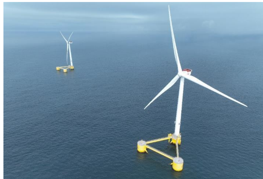
Figure 1 Example of a semi-submersible floating substructure. Photo of the WindFloat Atlantic project courtesy of Principle Power/Ocean Winds.
